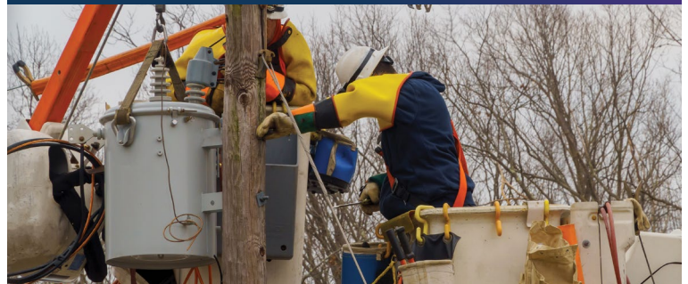
UTILITY ASSET INSPECTION
